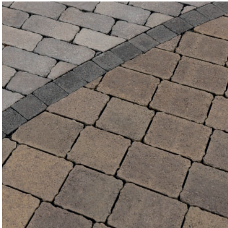
Permeable Concrete Block Paving
