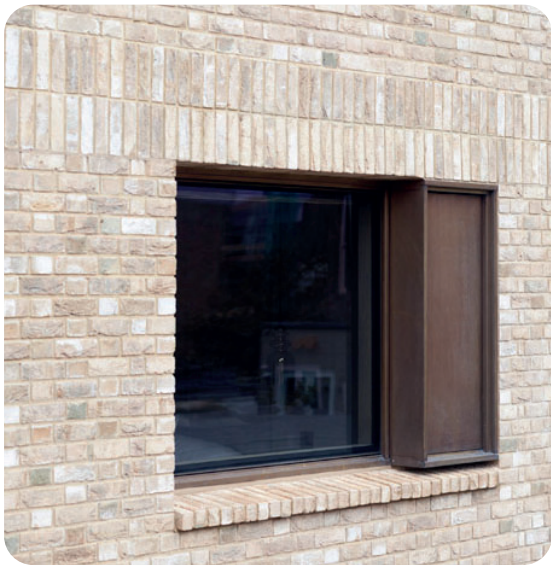
Architect: TDO Studio
