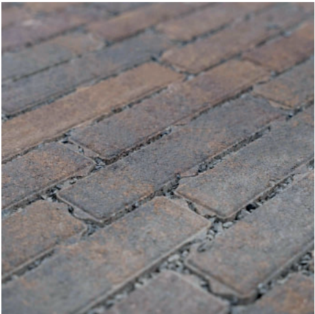
Permeable Feature Block Paving
